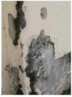
intercoat is peeling. Crazed paint is frequently recognizable by its thick and brittle surface.
